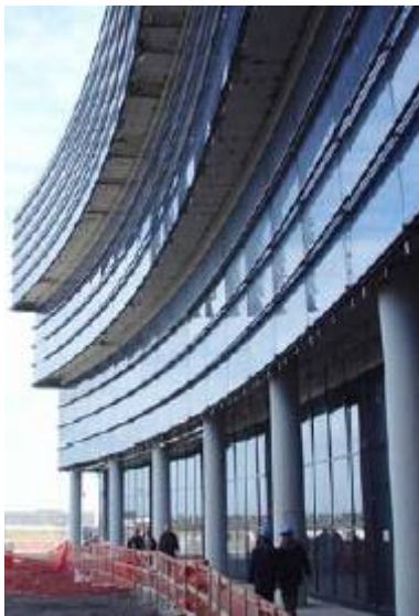
Exterior Façade During Construction
