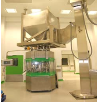
Servier UPA2 Facility, Arklow, Ireland
